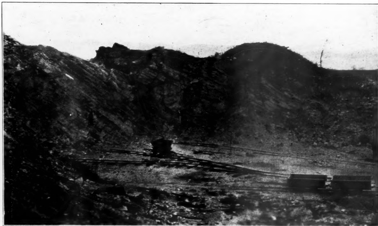
View of Quarry Tracks to Working Face and Chute from Upper Bench
